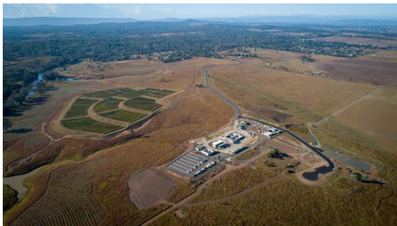
Figure 2 – Cedar Grove Wastewater Treatment Plant with associated wetlands and solar farm
