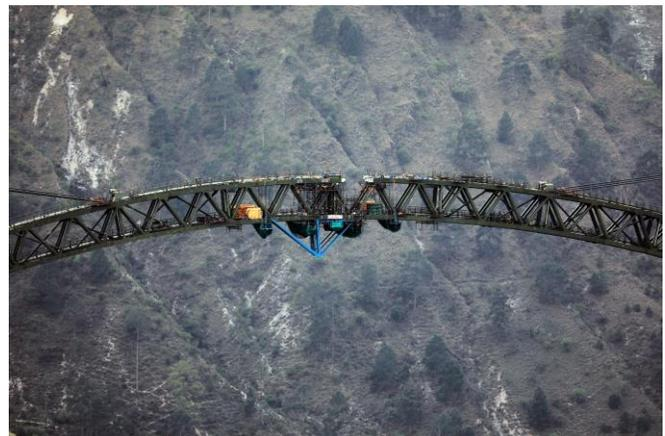
Figure 2 - Final moments before connecting the arch with engineers working on both levels of the arch
