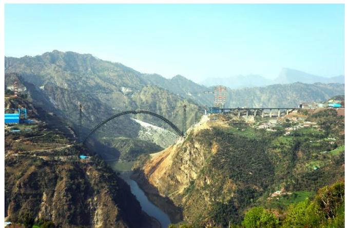
The image above shows the closure of the bridge's arch over the Chenab River in India — between Bakkal and Kauri in the Jammu and Kashmir region, in the northern part of India. The railway will be built over the arch.
