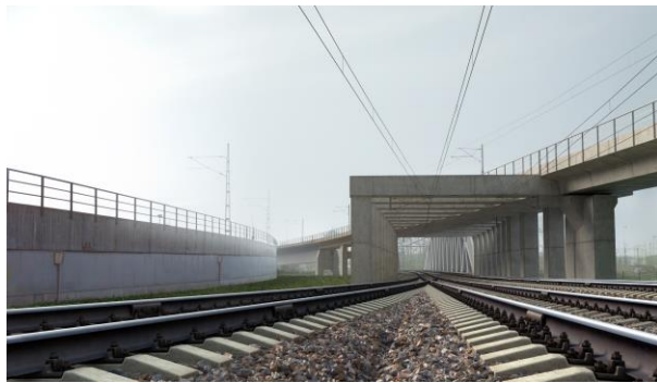
Photo: Trafikverket and Degree of Freedom The bridge is part of the Olskroken project in Gothenburg, Sweden. The project used alternative additives to decrease the amount of cement in the concrete bridges, supporting carbon-emissions reduction.
