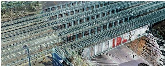
This WSP image represents the initial creation of a digital twin model of a rail bridge, utilizing a point cloud created from a terrestrial laser scan and site imagery. The model can be used for a variety of engineering and inspection purposes throughout the project lifecycle.
