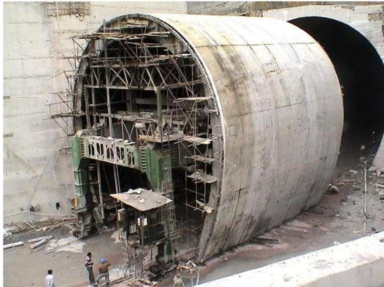
**Figure 1.** An impressive 15m high diversion tunnel lining shutter
