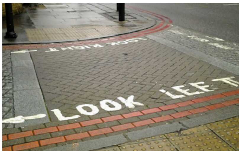
Image 4 – Tactile warning indicators and coloured pavers used to attract attention to crossing and instruction
