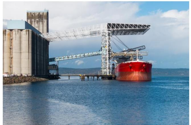
As an alternative, WSP has been working on a “Safe Haven” concept, whereby the entire berth is covered, providing fully enclosed ship loading operations. This is a relatively new concept in the marine terminal sector, one which has recently been implemented by Arcelor Mittal at North Port in Ghent. The scale is much smaller and targeted for coastal vessels and waterway barges handling breakbulk, however it is a concept that can be scaled up in the right conditions.
