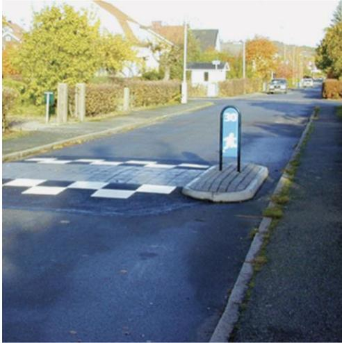
Figure 4 – speed hump on a local street in Gothenberg, Sweden
