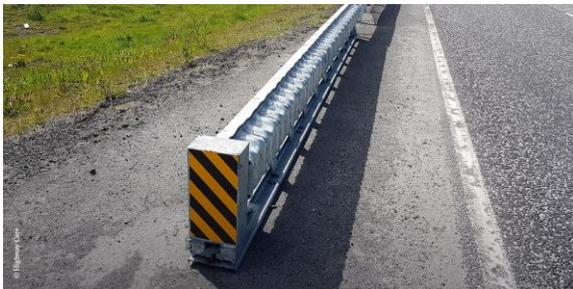
Figure 3 - Energy-absorbing barrier terminal (photo: courtesy of Highway Care)
