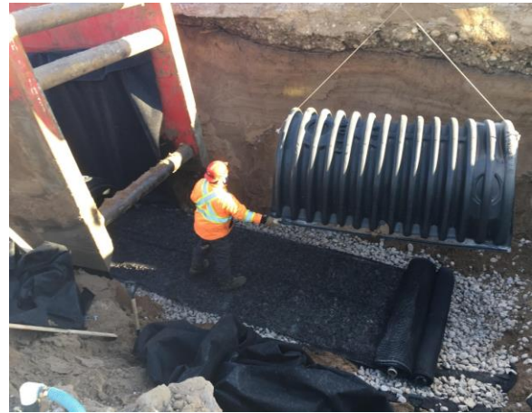
Figure 3 - Groundwater table conveyance system with geotextile grid installed underneath
