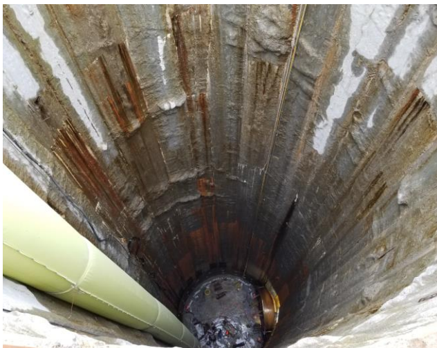
Figure 3 – TBM launch shaft
