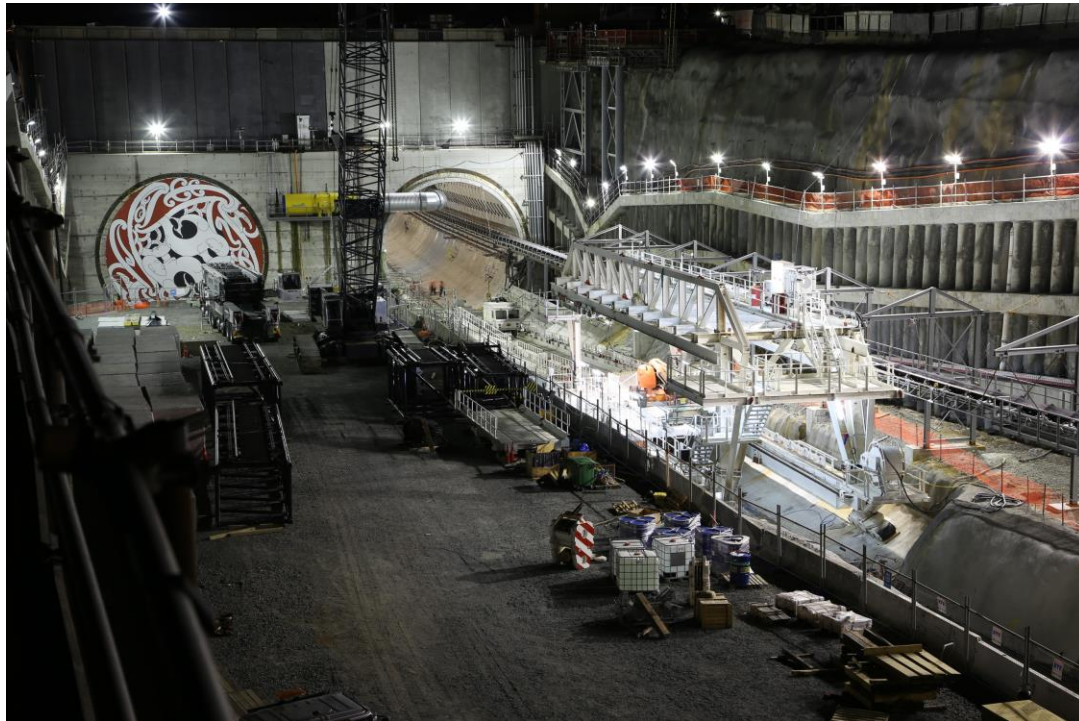
Image above: Waterview Tunnel, Auckland - courtesy of New Zealand Transport Agency
