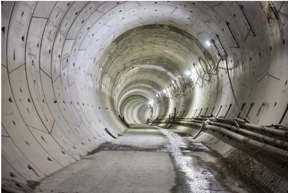
Figure 1- City Rail Link Karangahape Station Bored Tunnel, Auckland, New Zealand
