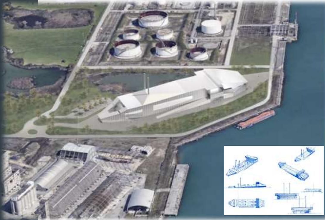
Design of a Waste to Energy (WTE) plant at Porto Marghera in Italy. The facility will treat a mix of dewatered and dried sludges from municipal wastewater treatment plants across the Veneto region. The WTE plant will produce electricity for self-consumption and the surplus will be released to the national network.
