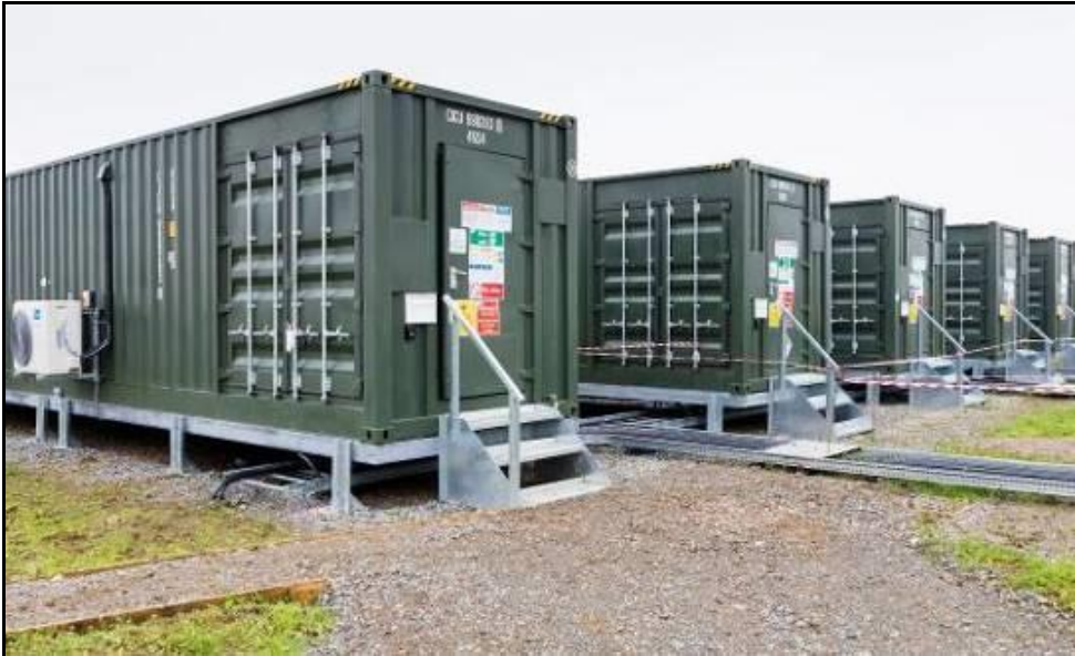
Photograph 1.2: Example of BESS located in storage containers
