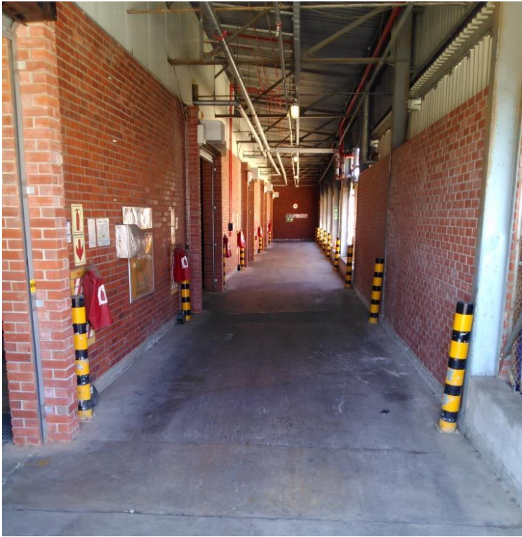
Figure 5. Outside corridor of the Flammable drum store from the left-hand side
