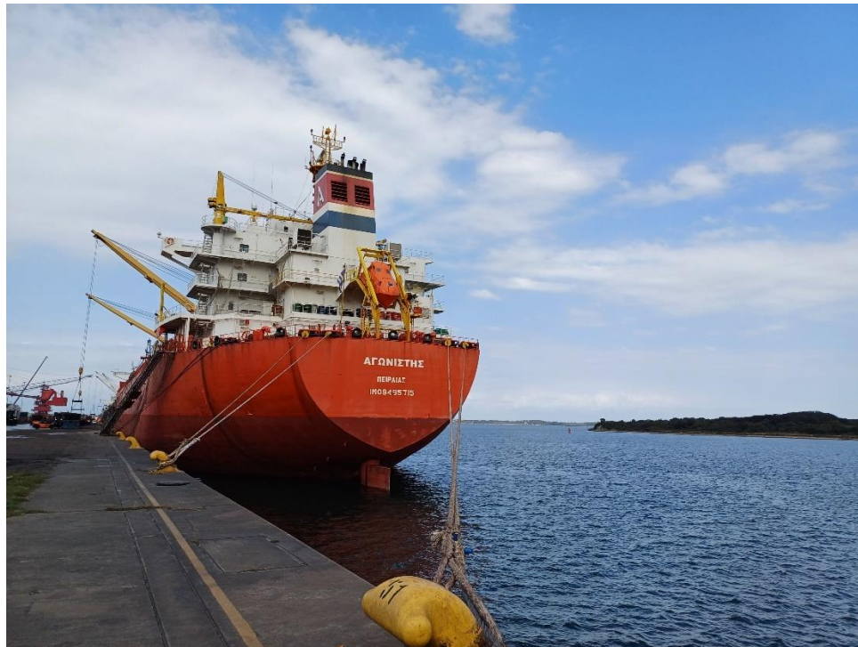
Bay area adjacent to the existing 600 series quay wall
