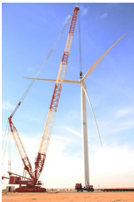
Figure 4-5: Crawler Crane used to assemble turbine (Liebherr, 2017)
