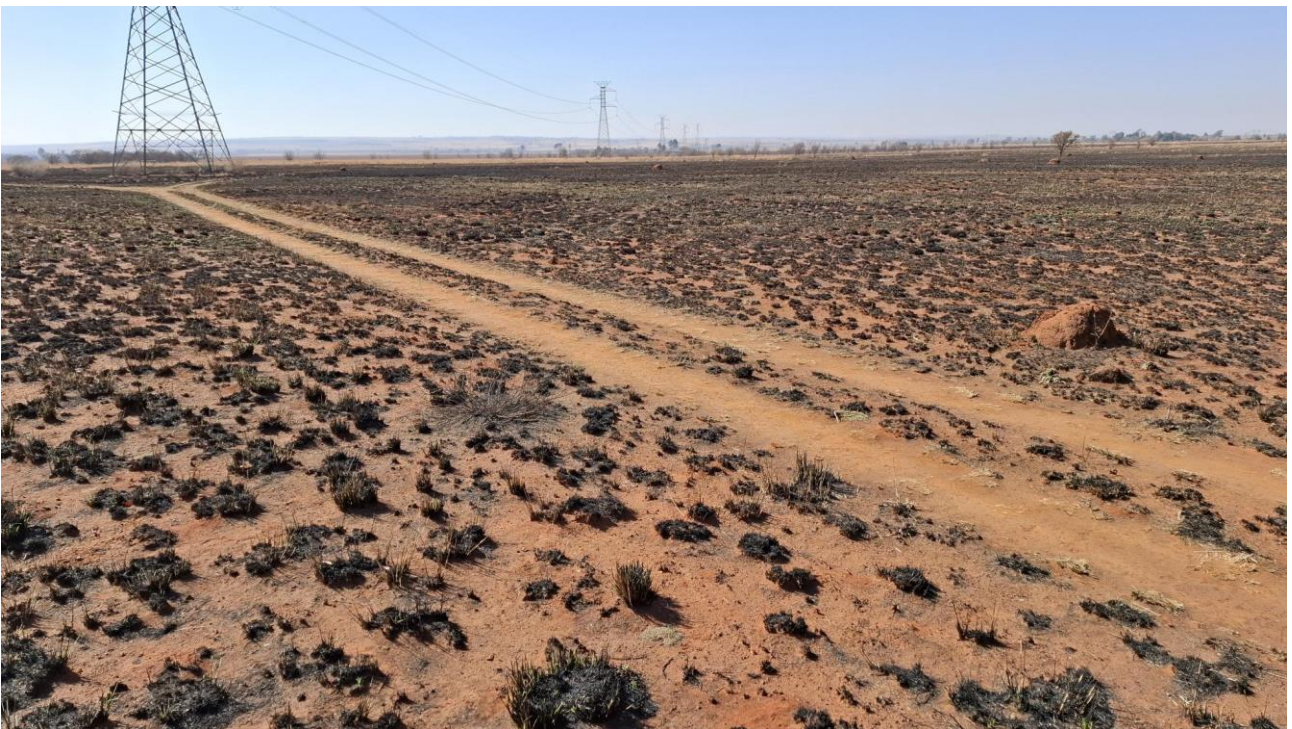
Figure 5. Typical site conditions.
