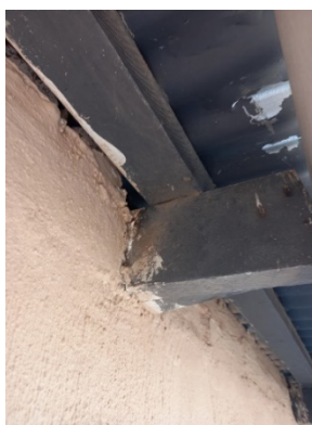
i) Kromhof – gap with smudgemarks in farmhouse roof
