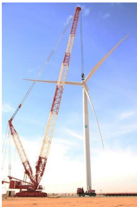
Figure 4-6: Crawler Crane used to assemble turbine (Liebherr, 2017)
