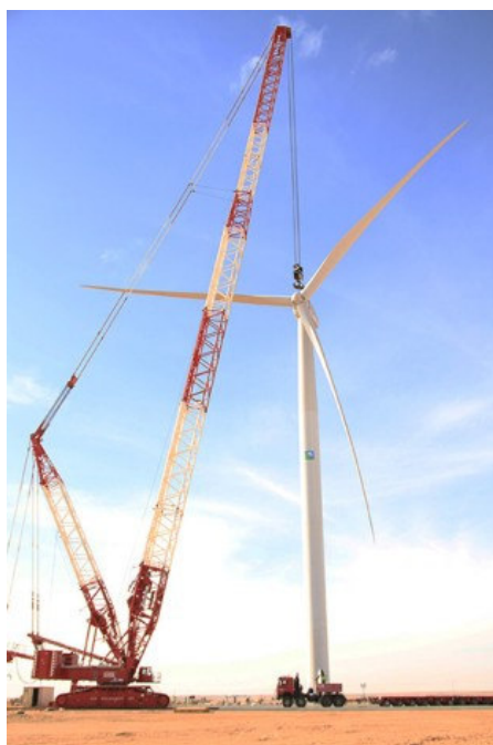
Figure 4-6: Crawler Crane used to assemble turbine (Liebherr, 2017)
