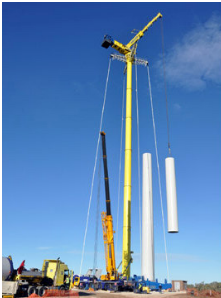
Figure 4-7: Cranes at work
