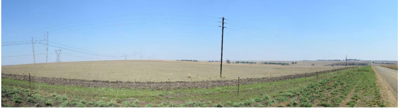
Figure 7-29 - High-mast power lines traverse parts of the project site
