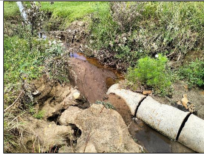
Representative photographs of the current condition of the seep wetland crossing to WTG 25 which requires immediate attention.
