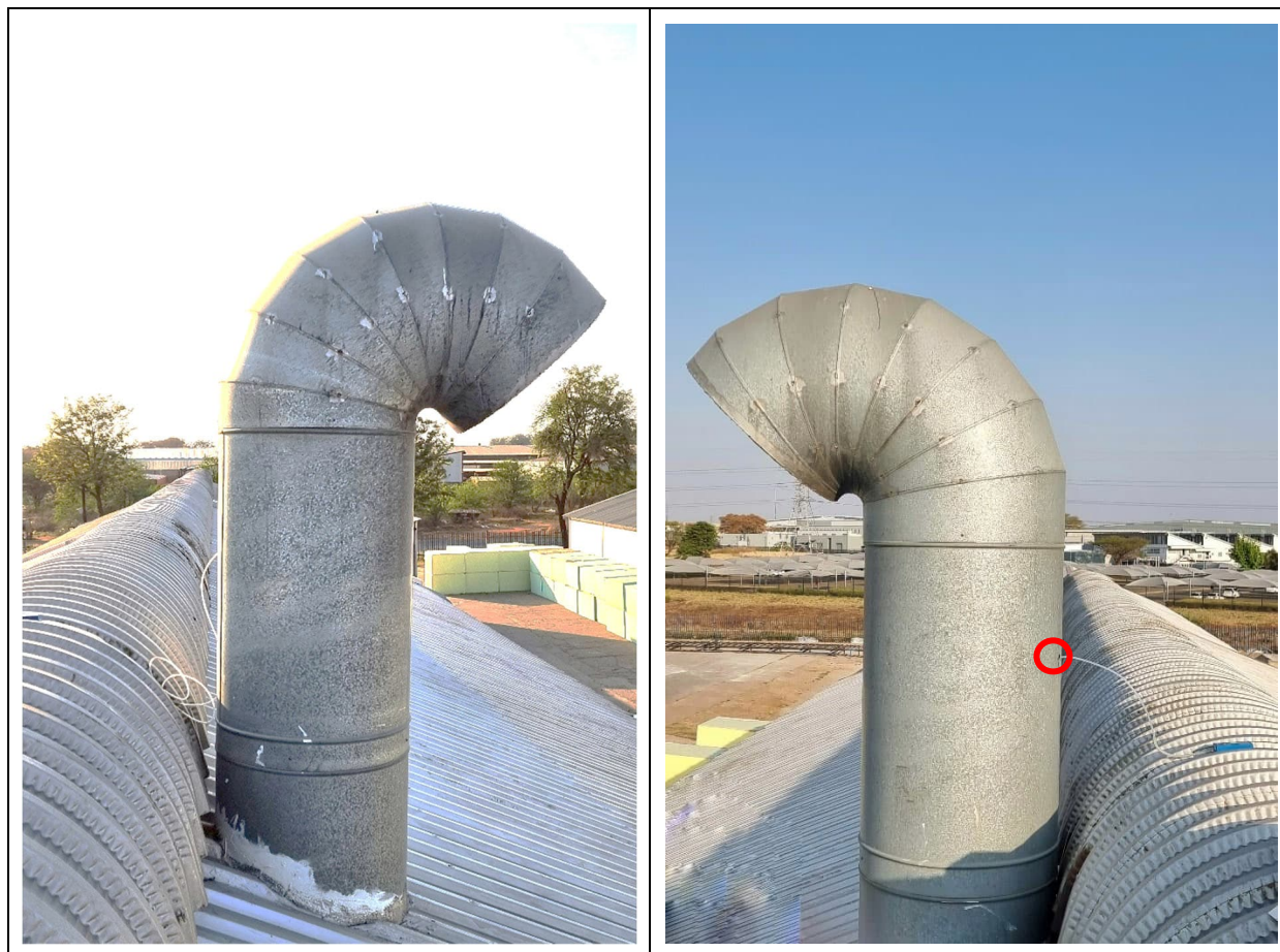
Figure 3: Two sources above the Extrusion Line. The source on the left is referred to as Front, as it is closest to the raw material feed section. The source on the right is referred to as the Back because it is closest to the finished foam section of the line. The sample points were in approximately the same location on each source and is highlighted with a red circle on the Extrusion source. Shown is the pump analyser setup. Pictures taken towards the East and West, respectively.
