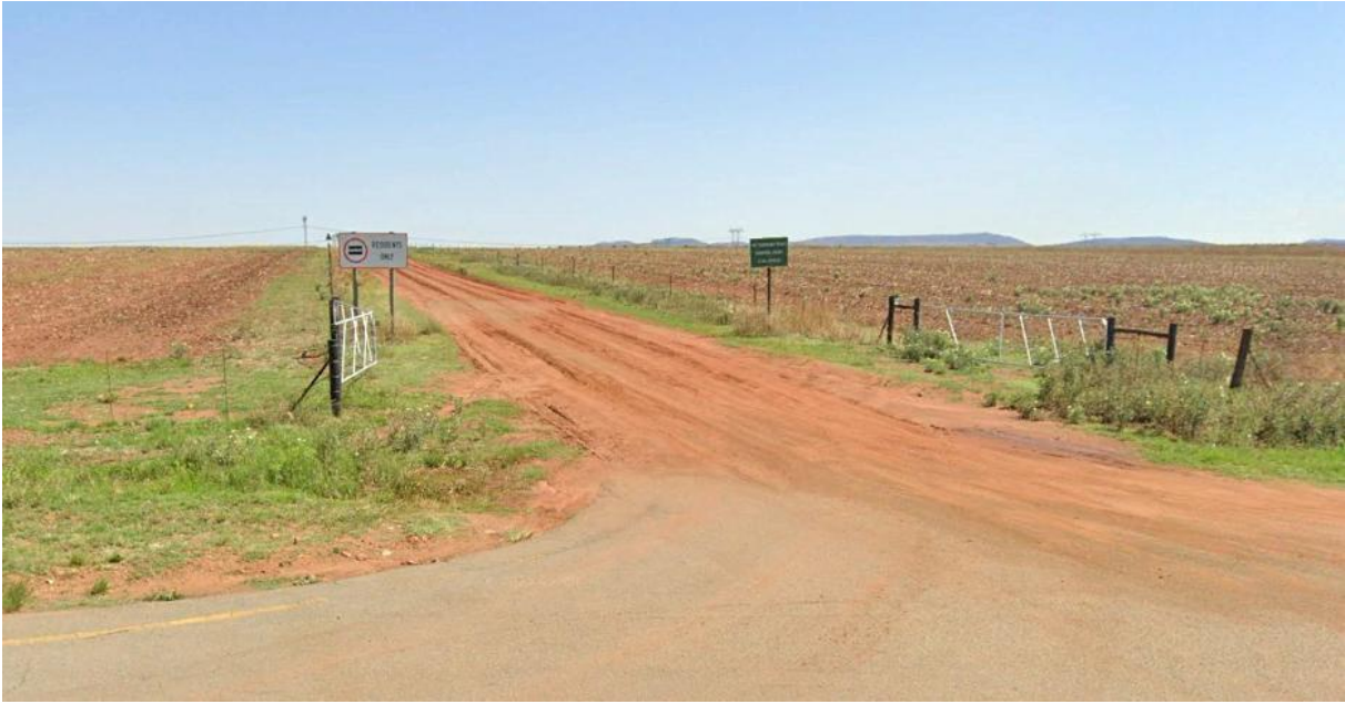
Figure 7-102 - View of existing access road (D1220) on P243/1
