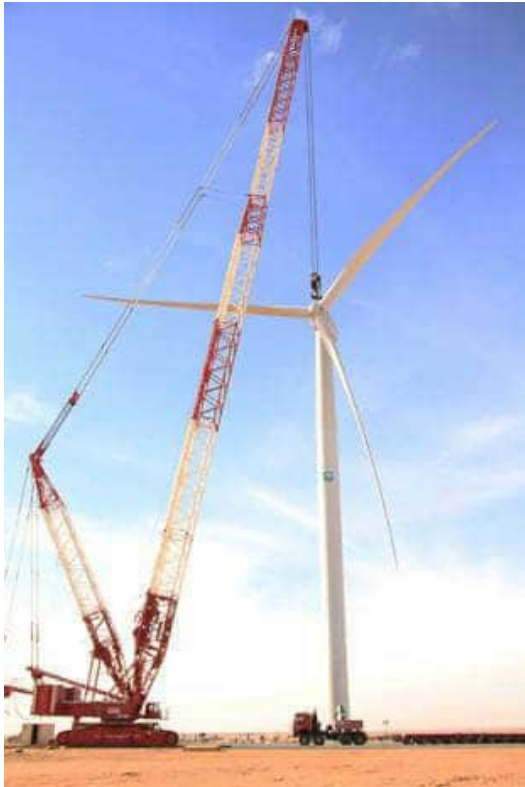
Figure 5-5: Examples of Crawler Cranes used to assemble turbines
