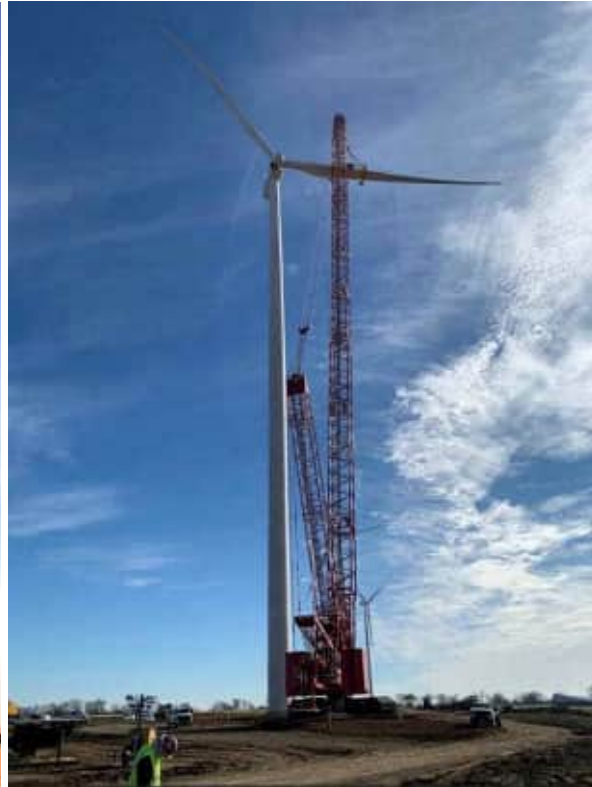
Figure 5-5: Examples of Crawler Cranes used to assemble turbines
