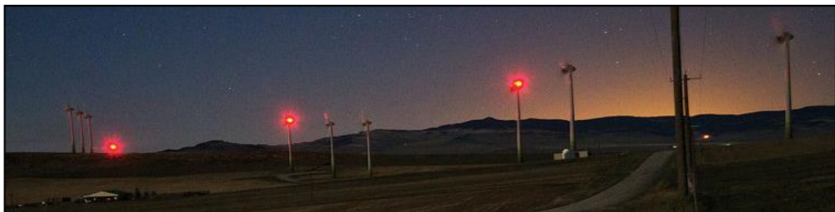
Figure 29: Aircraft warning lights fitted to the wind turbine hubs 12
