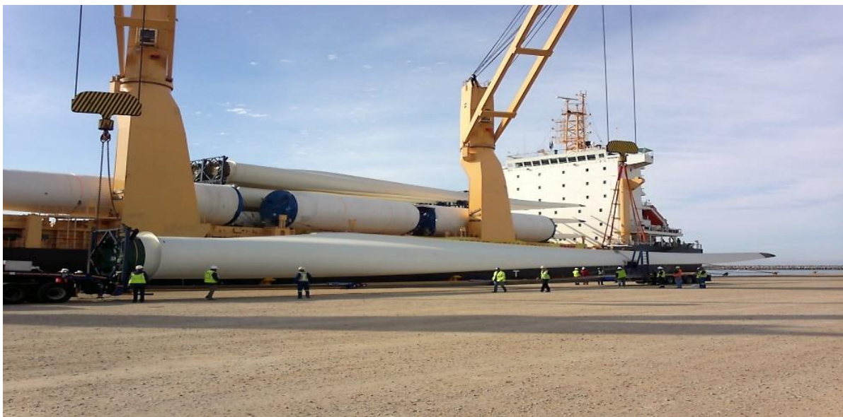
Figure 5-6: Cranes at Port of Entry (Authors picture)
