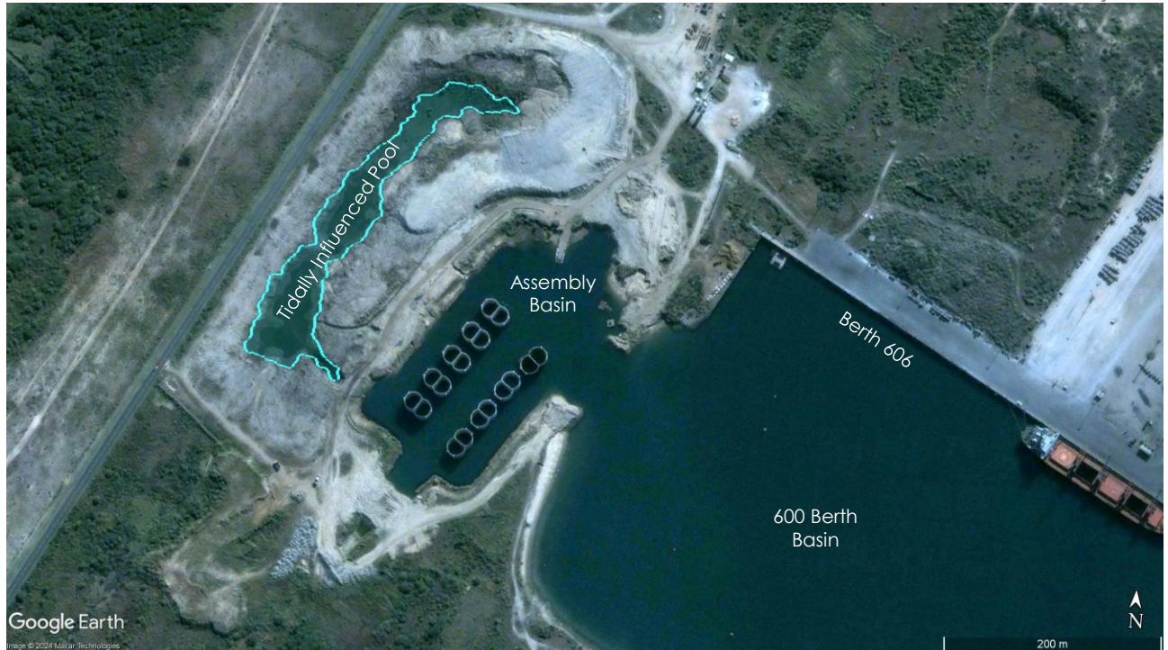
Figure 6-26 - Aerial view of caissons in the Assembly Basin in the 600 Berth Basin in the Port of Richards Bay. The berm that sealed the basin has been breached in preparation of caisson floating to Berth 306. The existing tidally influence pool referred to in the text is highlighted.
