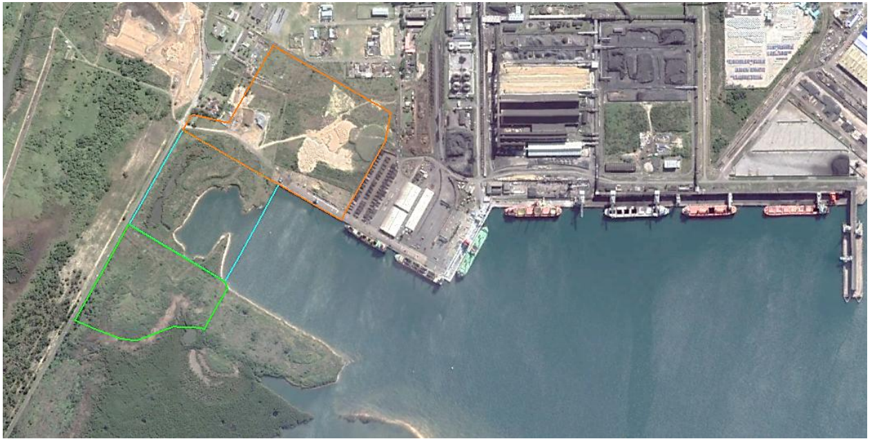
2015 Compensation area and berth basin (green and blue) show signs of recovery while there is ongoing materials storage and handling within the container footprint. Note start of mangrove development within the tidal pool and woody vegetation developing within compensation area
