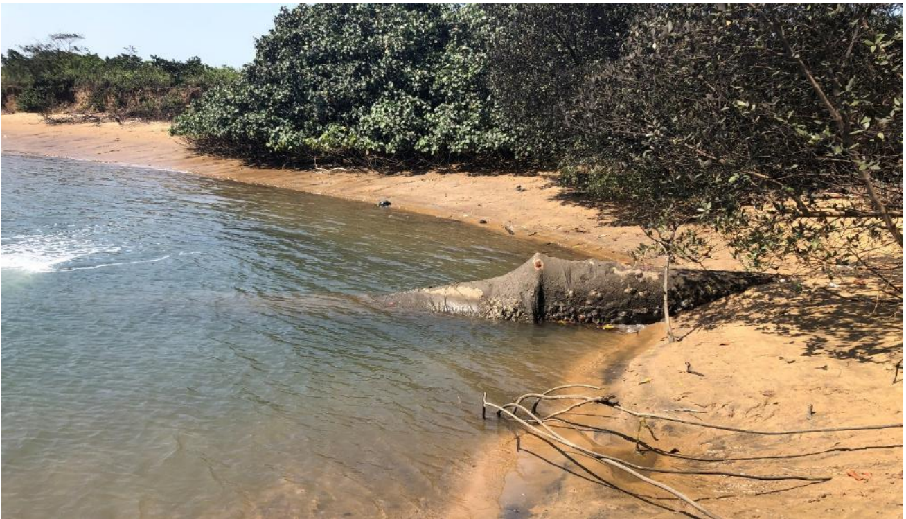
Fig. 9. The pipeline apparently allowing tidal flow between the mangrove stand in the Berth 605 project footprint and the harbour.
