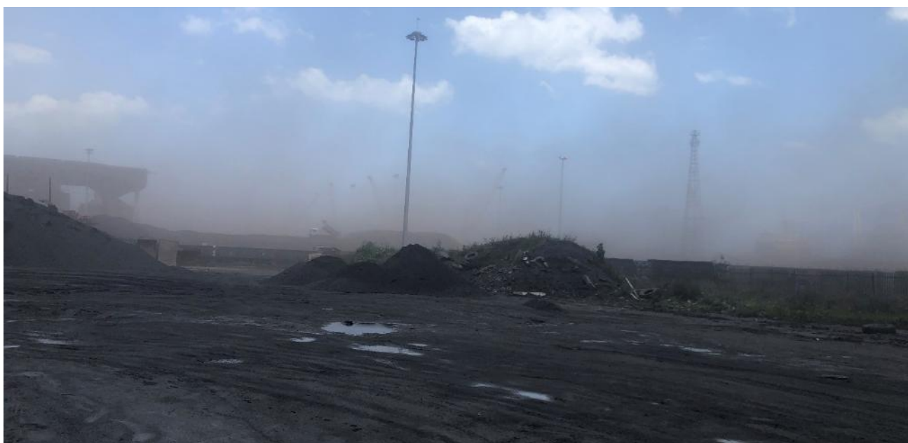
Fig. 13. Coal and other dust associated with heavy truck traffic in the Berth 605 project area under strong-wind conditions.
