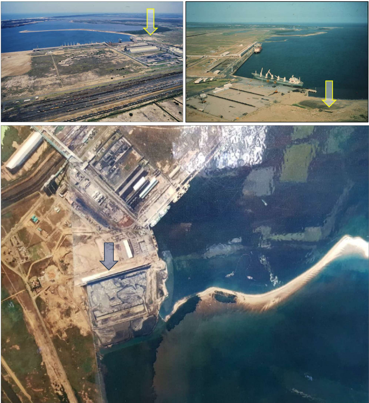
Figure 12. Aerial views of the Port of Richards Bay before and during construction of the 600 Berth Basin (position shown by arrows).
