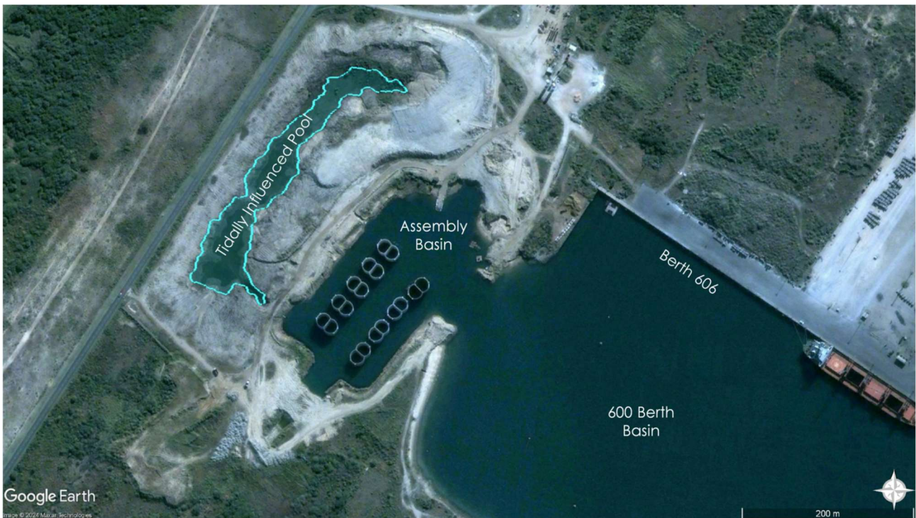
Figure 15. Aerial view of caissons in the Assembly Basin in the 600 Berth Basin in the Port of Richards Bay. The berm that sealed the basin has been breached in preparation of caisson floating to Berth 306. The existing dimensions of the tidally influenced pool referred to in the text is highlighted.
