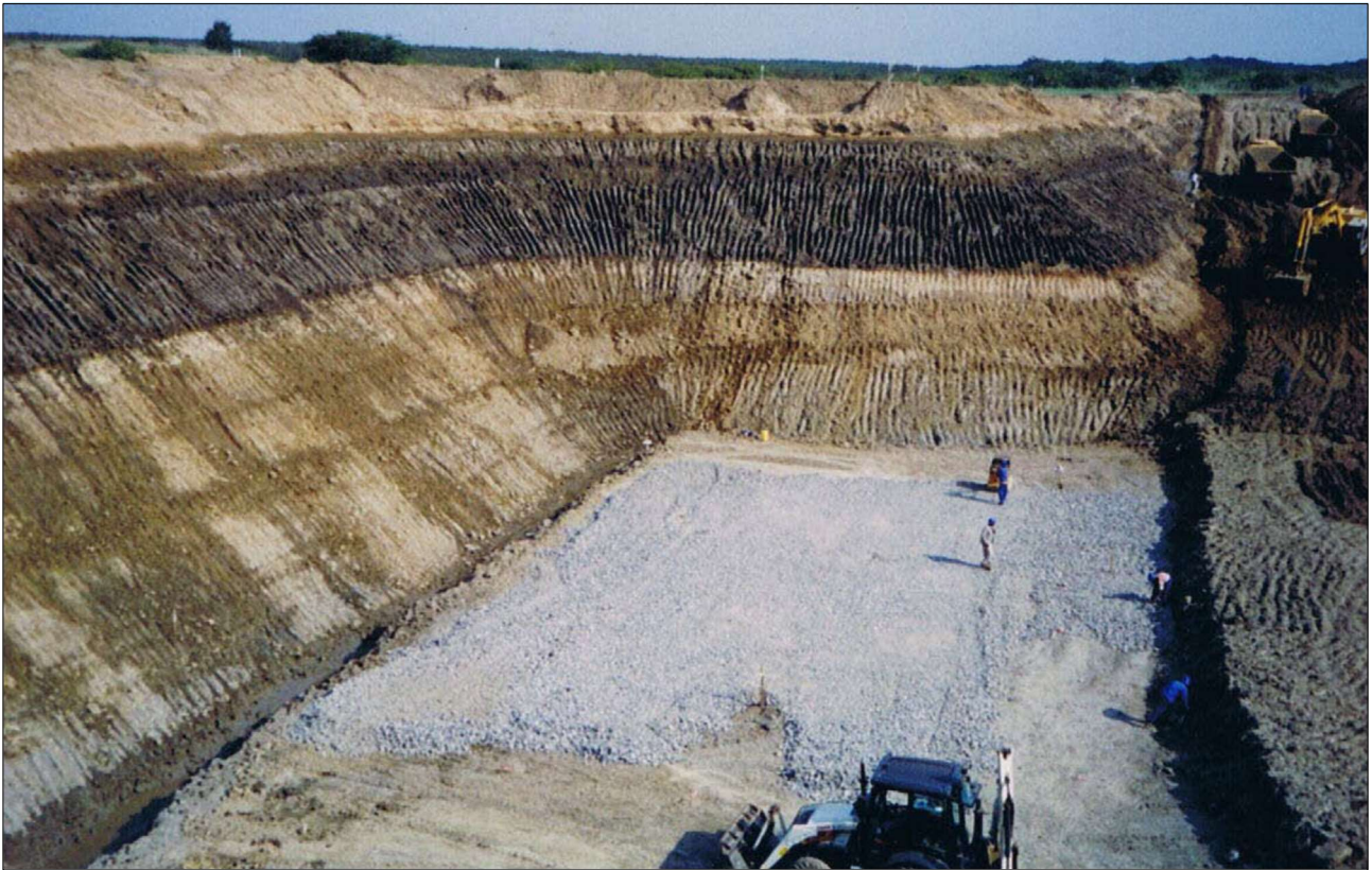
Figure 19. Photograph of the Assembly Basin in the 600 Berth Basin in the Port of Richards Bay, showing geological formations in the area. Photo from Albert van Jaarsveld.
