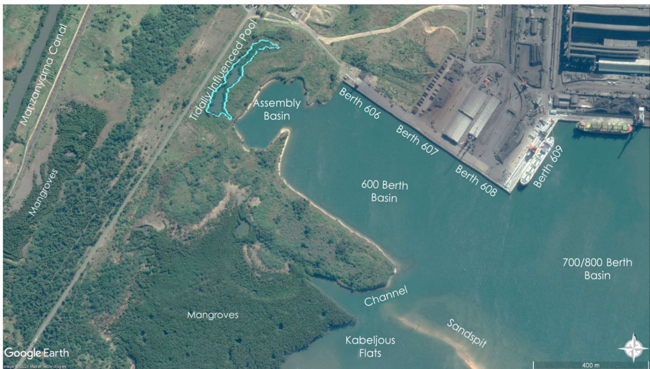
Figure 11. Aerial view of the 600 Berth Basin and its surrounds in the Port of Richards Bay.
