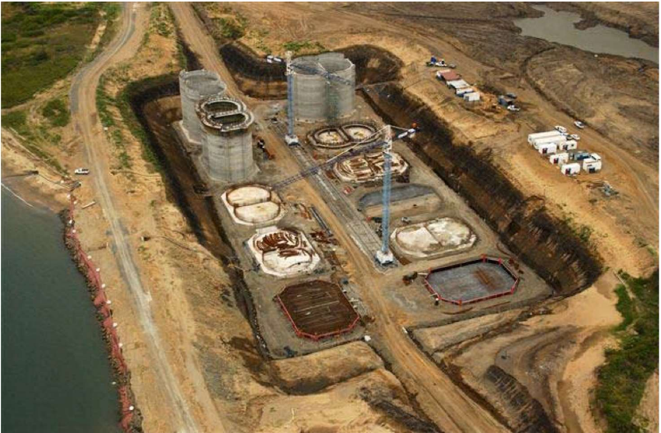
Figure 14. Aerial view of caisson construction in the Assembly Basin in the 600 Berth Basin in the Port of Richards Bay. Part of the existing tidally influenced pool referred to in the text is visible in the background. Photo from Albert van Jaarsveld.
