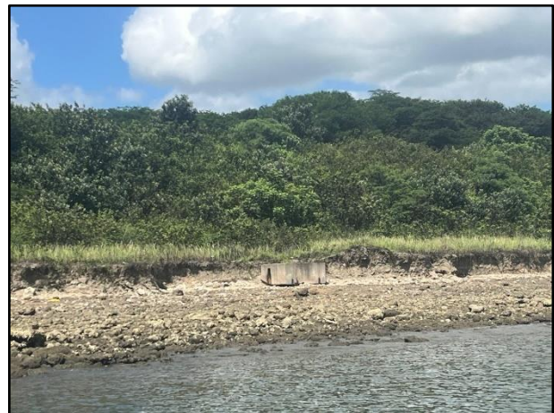
Figure 13: Concrete block in the intertidal zone
