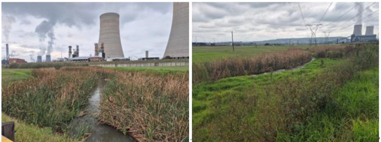
Figure 5-10 - Photographs illustrating CVB2 characteristics and conditions in 2026: (Right) the main channel of the Groot-Bossiespruit with T. capensis and P. australis along the channel, (Left) the AIP infestation along the northern edge of the system
