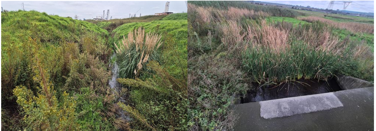
Figure 5-6 – A highly transformed watercourse crosses the site from north to south and exits underneath an embankment through a concrete culvert
