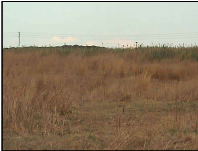
Figure 39 Reeds SCS(E) PC dam wall
