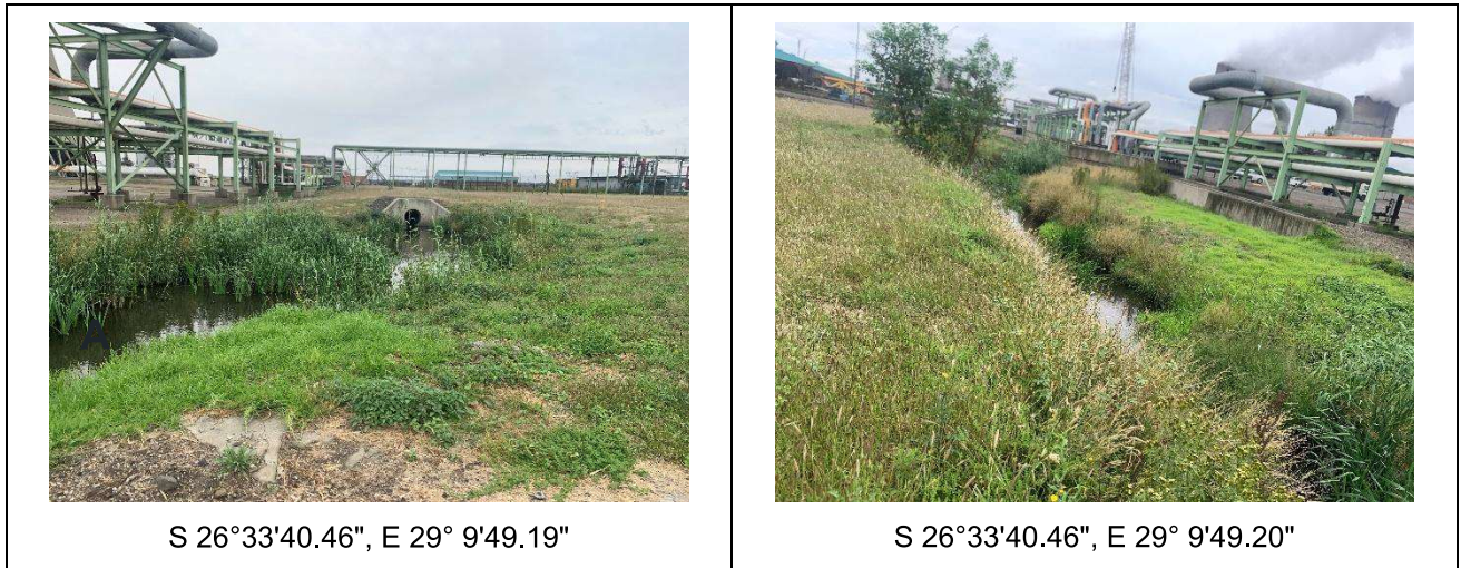
Figure 7-2 - Field survey images of the MRG Pipeline route
