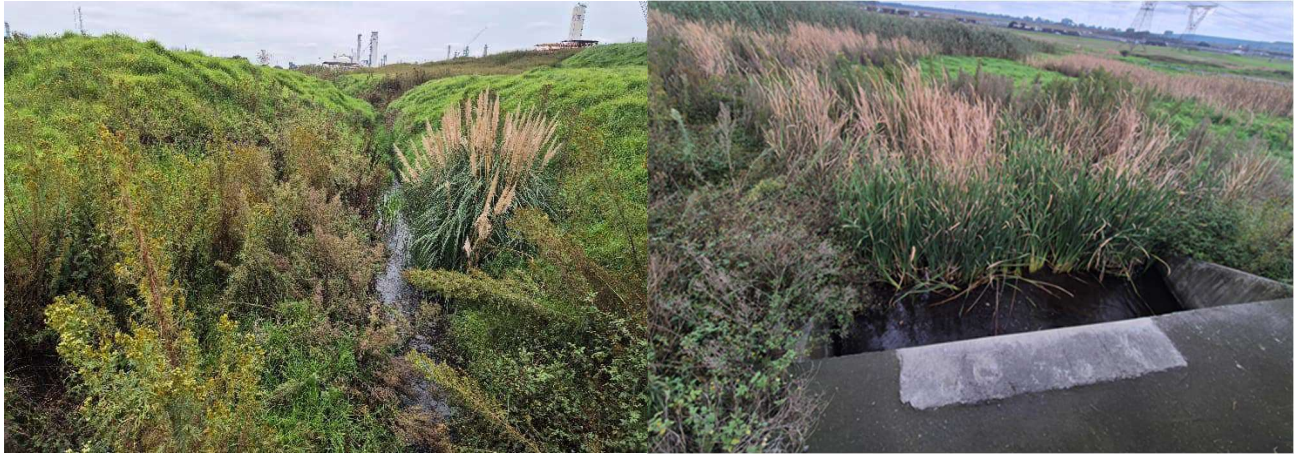
Figure 5-3 – A highly transformed watercourse crosses the site from north to south and exits underneath an embankment through a concrete culvert
